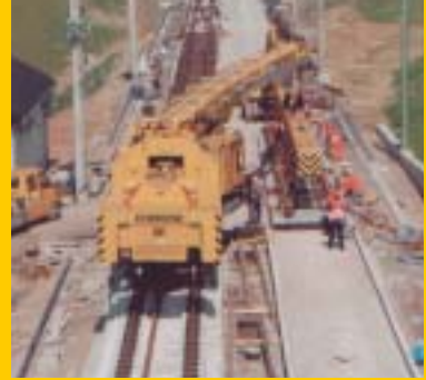
Installation of a high speed turnout.
