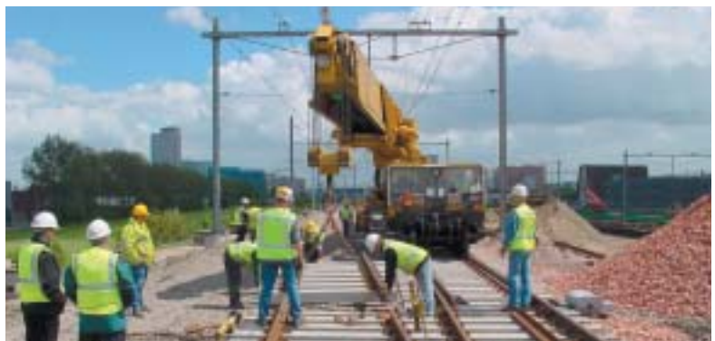
Installation of a turnout.
