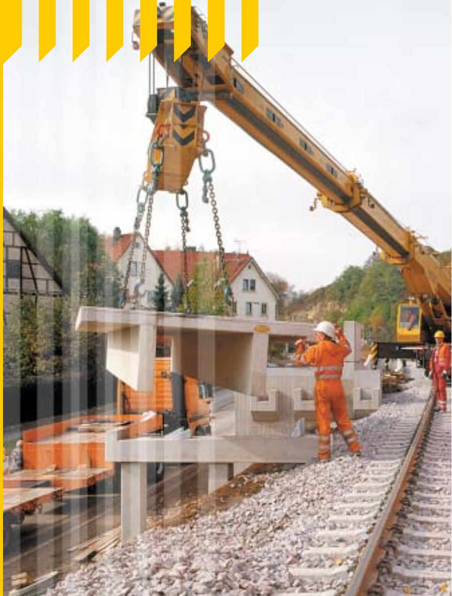
Installation of precast concrete parts within the working clearance diagram.
