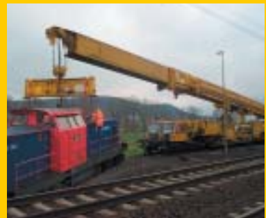
Recovery of a derailed loco.
