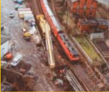
Installation of a temporary bridge within the working clearance diagram.
