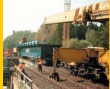
Tandem lift to install a 120 t steel bridge.
