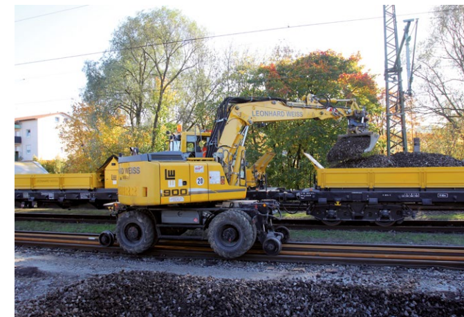
▲ Loading with excavated material under catenary line
