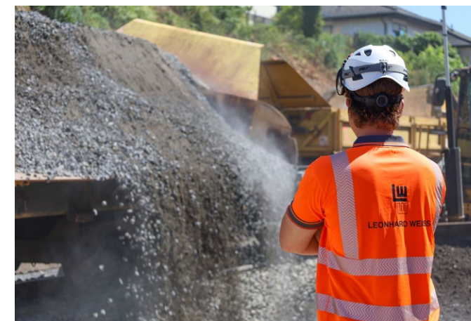
▲ Site of unloading of excavated material
