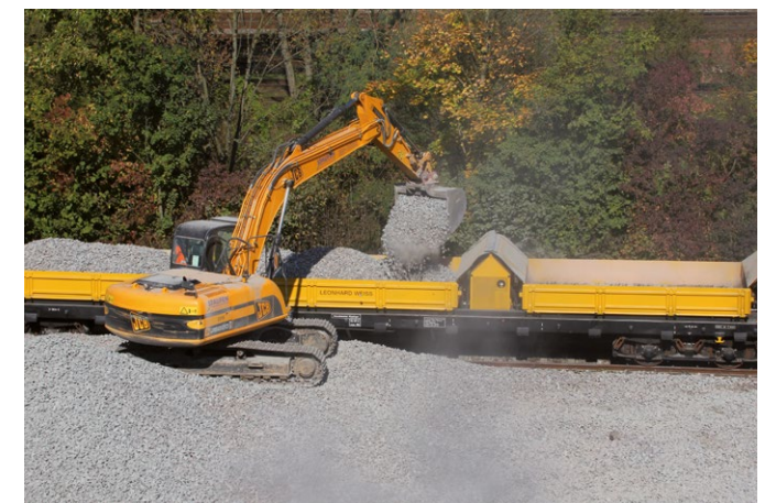
Loading with new ballast ▲
