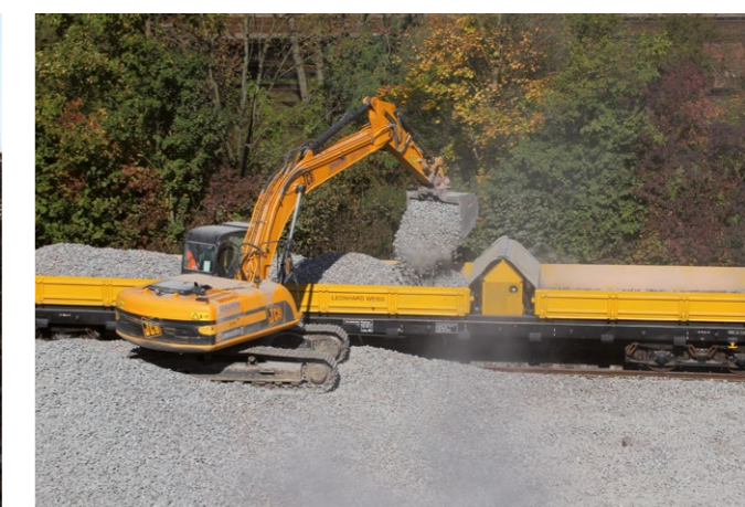
▲ Loading with new ballast ▲
