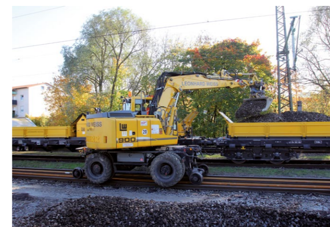
▲ Loading with excavated material under catenary line
