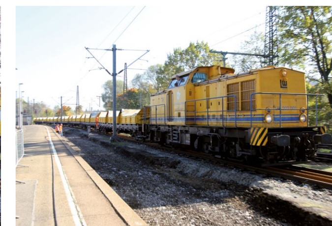
▲ Transport to site of unloading ▲
