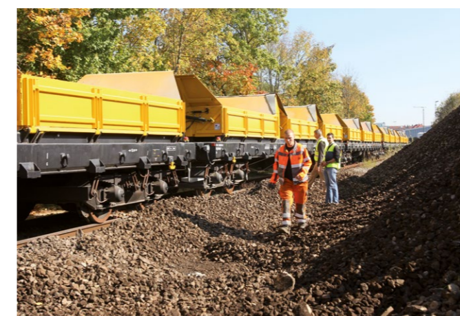
▲ Site of unloading of excavated material
